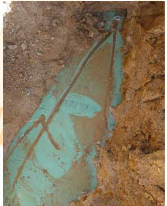
Pipeline protective coating damaged by a backhoe
