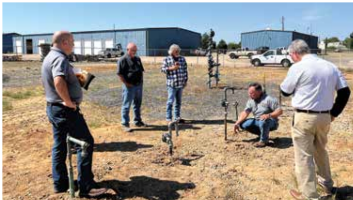
CenterPoint Energy leak city.
