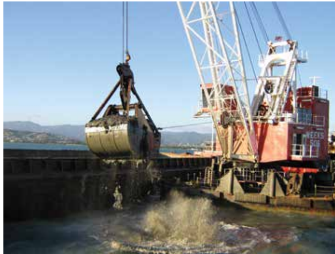
Weeks Clamshell at Tappan Zee Bridge, NY
